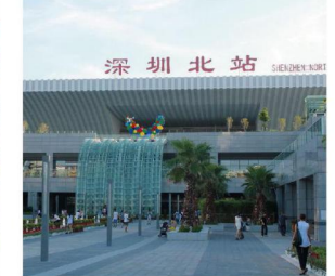
Shenzhen North Railway Station
