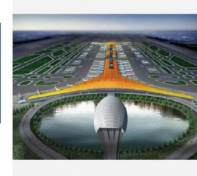
Beijing Capital airport- T3 terminal
