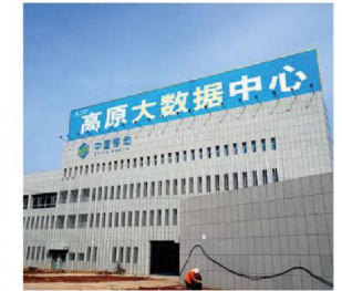
China Mobile data center
