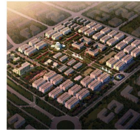
China Telecom data center
